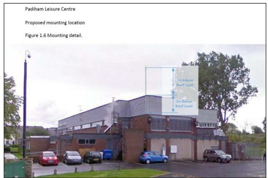
The mast would project 7m above roof level, being attached at a street frontage corner of the building by a 3m high bracket arrangement affixed externally to the upper, cladded wall of the building. The mast would have a width of around 9cm.
